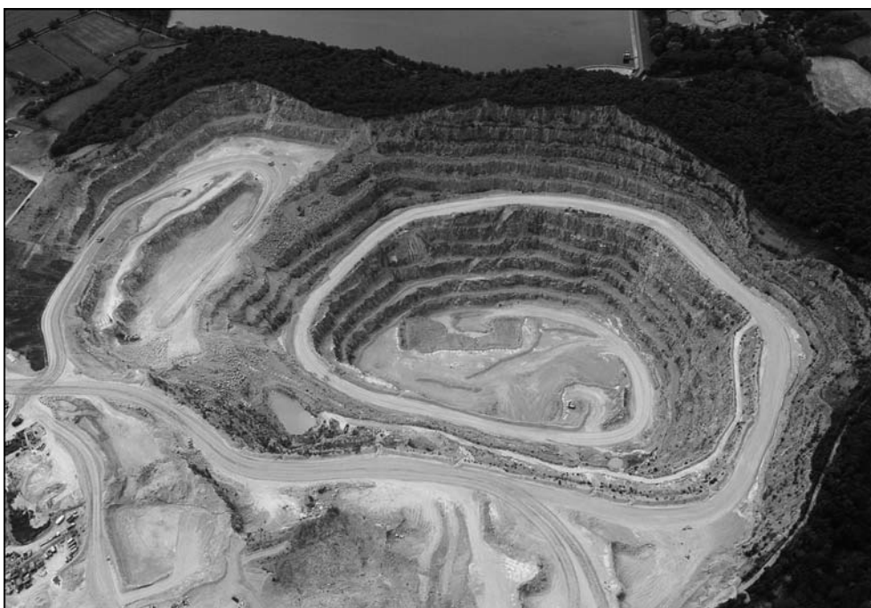
Figure 15. Aerial view looking southwest over the active Buddon Wood Quarry, Mountsorrel, in May 2005. Swithland Reservoir can just be seen at the top of the picture. (Photo: Lafarge Aggregates)
