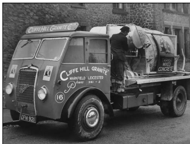
Figure 26. Cliffe Hill Granite Company truck delivers mixed concrete. (Photo: MQP)
