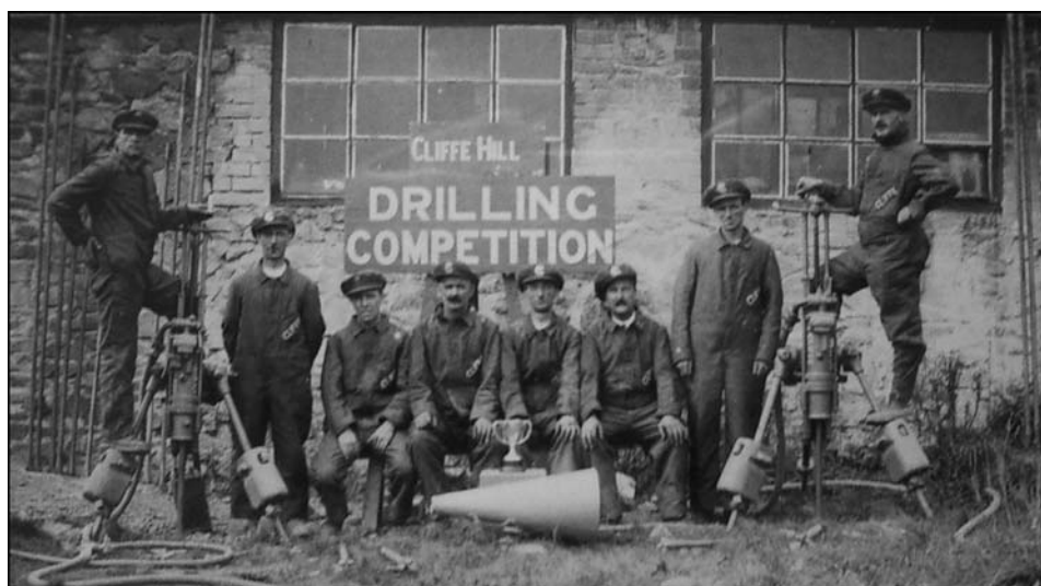
Figure 17. Drilling competition at Old Cliffe Hill Quarry. (Photos: MQP)
