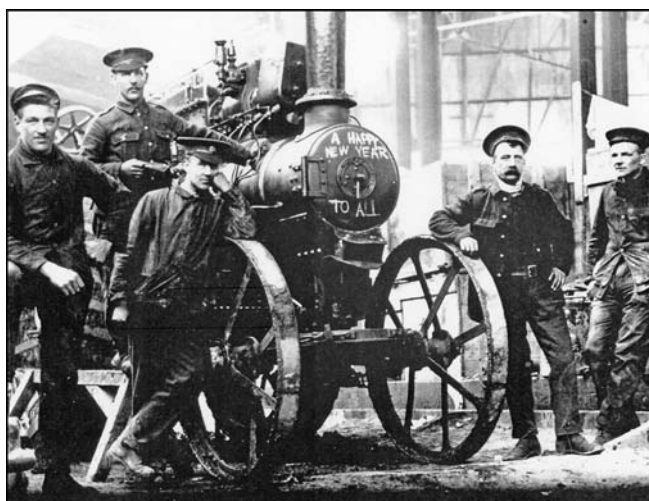
Figure 25. New Years Day 1915, at Whitwick Quarry, with seasonal greeting written on the front of the steam engine. Origins of this photograph are unknown, but it is thought that it could be either soldiers requisitioning a steam lorry from Whitwick Quarry, or former quarrymen visiting the quarry on leave. (Photo: Whitwick Historical Group)
