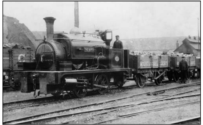
Figure 14. The Baron and wagons loaded with granite, Mill Yard, Mountsorrel Quarry, c1900. Note the engine shed in the background(Photo: Lafarge Aggregates)
