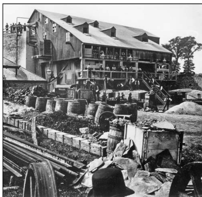
Figure 12. The crushing mills, known as the High Level at Mountsorrel Quarry, with curious workforce looking on, c1880. The barrels are filled with crushed granite, ready for distribution. (Photo: Lafarge Aggregates)
