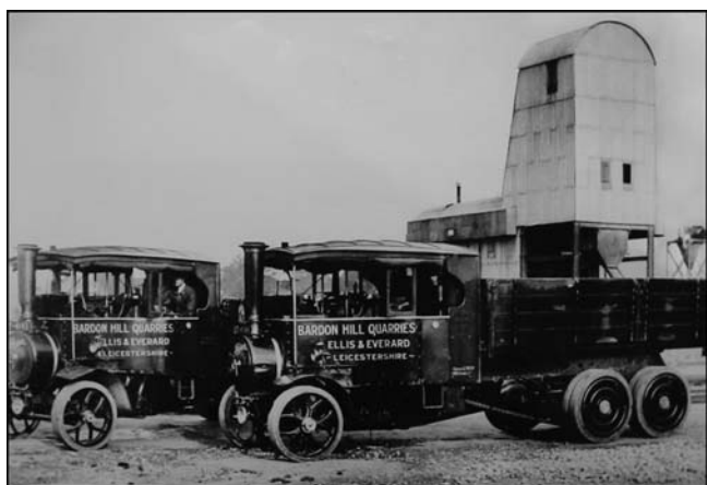
Figure 9. Ellis & Everard's steam lorries at Bardon Hill Quarry, c 1920. (Photo: Aggregate Industries Archive)
