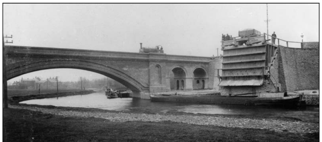
Figure 13. The bridge at Mountsorrel, c 1870, with a locomotive on it. Right of the bridge are the loading chutes, with side-tip wagons on top feeding aggregate to barges on the canal. (Photo: Lafarge Aggregates)
